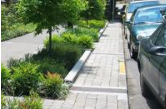
Advance Streetscape and Public Realm Projects
