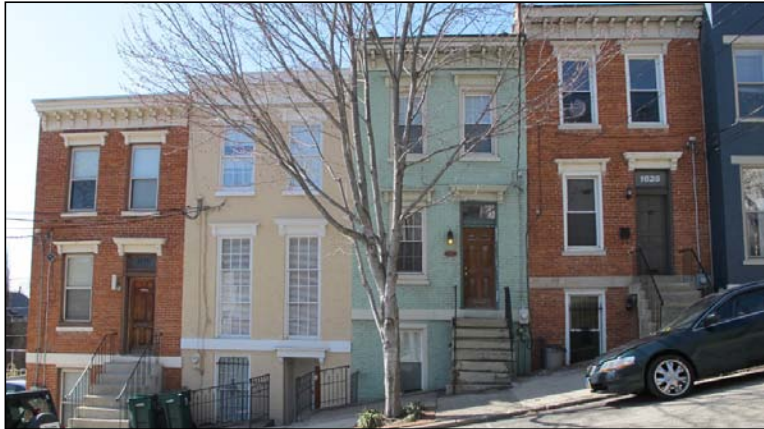
Classically detailed brick Rowhouses are stepped down a steep sidewalk.
