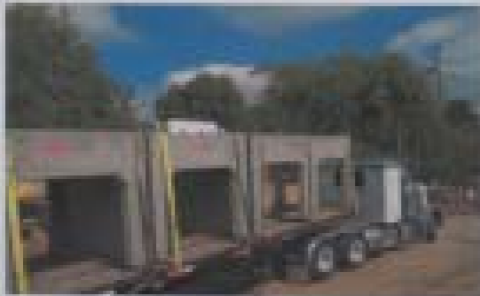
Two large concrete vaults have been installed to capture water from the city's mainlines. The concrete was made up of reusable units shown here during installation.
