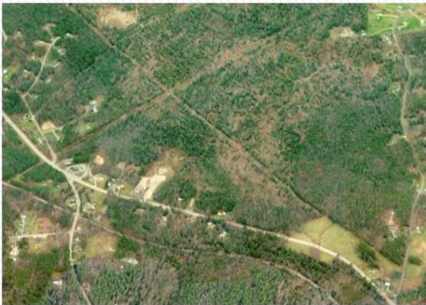
Emerging Strip at Rt. 196 & River Rd., Topsham
