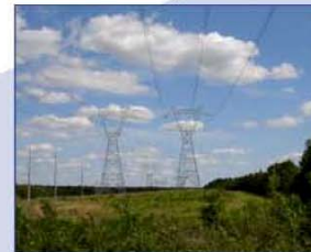
Major utility corridor slices through Planning Unit IV
